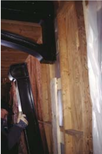
Figure 4. With the steel arch in its final position, the crew slipped the matching columns into place at each end (above), then bolted the mating members together (above right). A tapered drift pin helped line up the predrilled holes in steel components so it was easier to insert the bolts (far right). On the back, a \frac{3}{8} -inch-thick reinforcing plate joined the beam and column (right).
