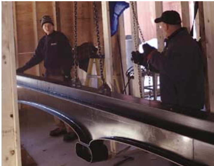
Figure 3. After notching the existing girder (far left), a carpenter slid a custom hanger into place to support both sides of the notch (left). The hanger was exactly sized to receive the new steel beam, which was chain-hoisted into place (below). Welded-on lifting points (below left) made the process easier and safer.
