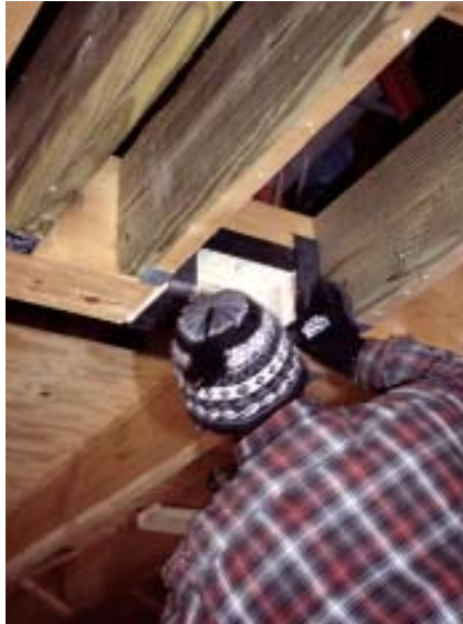
Figure 3. After notching the existing girder (far left), a carpenter slid a custom hanger into place to support both sides of the notch (left). The hanger was exactly sized to receive the new steel beam, which was chain-hoisted into place (below). Welded-on lifting points (below left) made the process easier and safer.
