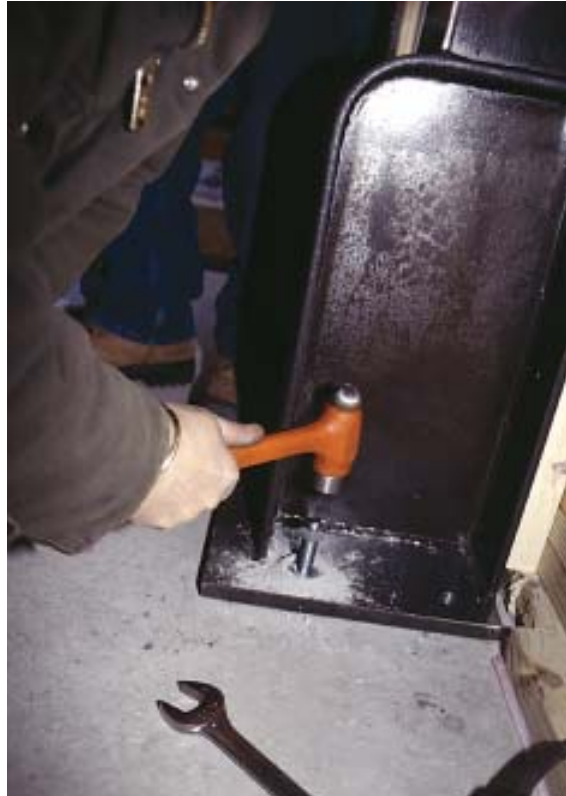
Figure 5. A rotary hammer (above left) made quick work of holes for the wedge anchors (above) that secure the column bases to the slab. Steel shims of various thicknesses (left) made up for irregularities in the concrete.
