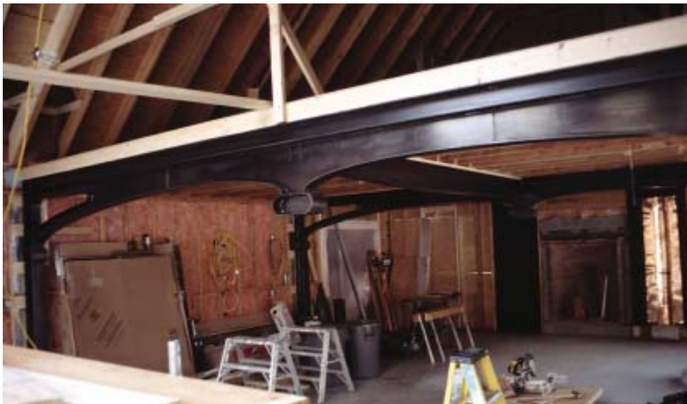
Figure 1. To transform this garage (left) into living space with an open floor plan, the author replaced the existing steel I-beam and supporting column with a framework of custom-fabricated decorative steel (below).
