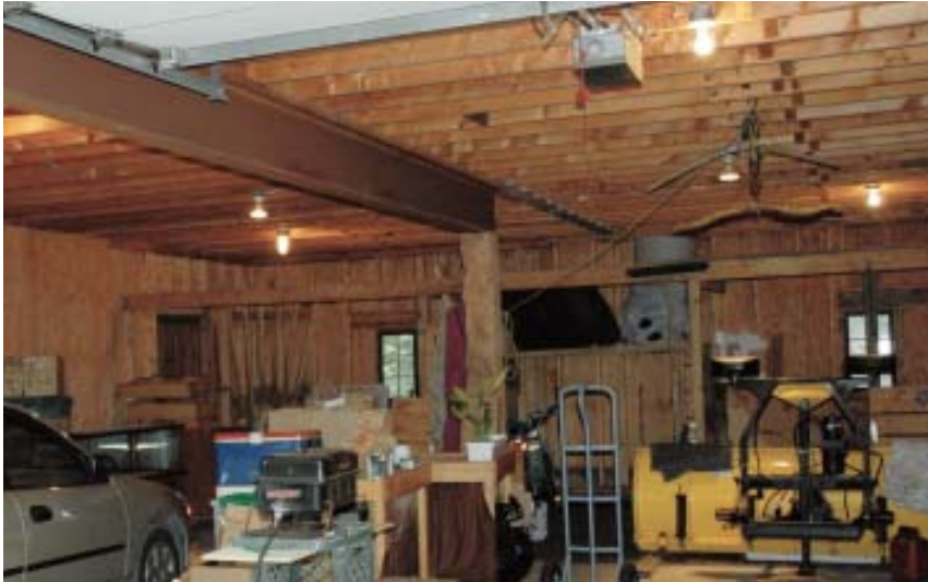
Figure 1. To transform this garage (left) into living space with an open floor plan, the author replaced the existing steel I-beam and supporting column with a framework of custom-fabricated decorative steel (below).
