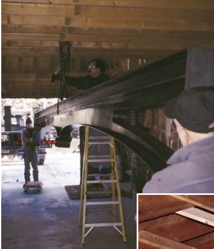
Figure 2. A three-ply 2x8 beam resting across the roof collar ties supported the chain hoist (left) used for lifting the steel beams. The author doubled up the collar ties (below) and beefed up the rafter connections with 1/2-inch bolts to handle the temporary load.
