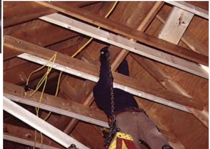
Figure 2. A three-ply 2x8 beam resting across the roof collar ties supported the chain hoist (left) used for lifting the steel beams. The author doubled up the collar ties (below) and beefed up the rafter connections with 1/2-inch bolts to handle the temporary load.
