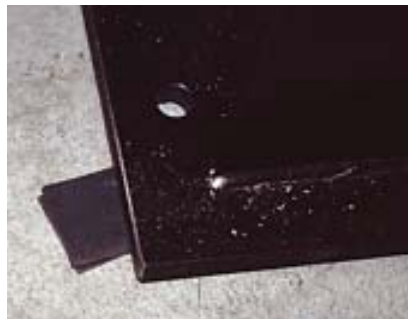
Figure 5. A rotary hammer (above left) made quick work of holes for the wedge anchors (above) that secure the column bases to the slab. Steel shims of various thicknesses (left) made up for irregularities in the concrete.
