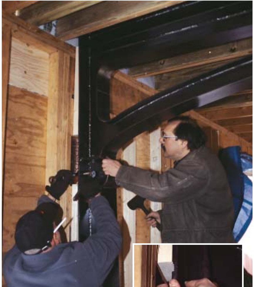
Figure 4. With the steel arch in its final position, the crew slipped the matching columns into place at each end (above), then bolted the mating members together (above right). A tapered drift pin helped line up the predrilled holes in steel components so it was easier to insert the bolts (far right). On the back, a \frac{3}{8} -inch-thick reinforcing plate joined the beam and column (right).
